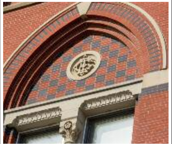
Restoration of painted brick
