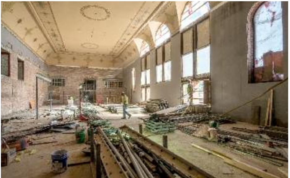
Corbett Tower Renovation
